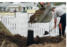
**Step 4** Remove Safety Top along scribed line and fill with concrete to desired height.
