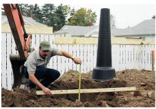
**Step 2** Install in desired location. (centre and Level on Safety Top)
