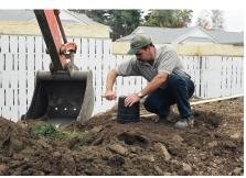
When required the FTB30 can be installed under the 8" and 10/12" Footing Tube (adds 90% more load bearing area)
